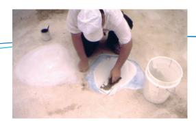
**Poxofill** can be used for permanent patching of concrete for a strong, lasting bond. Also used for anchoring diving boards, ladders and resetting tile.
