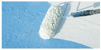
Rolls easily to transition your pool to allow an epoxy finish.
